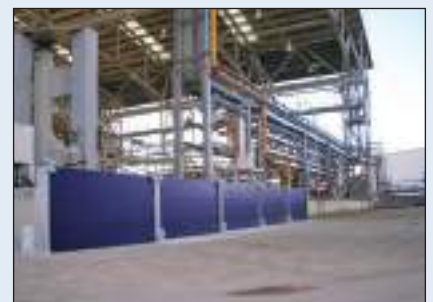
Multi-span 900mm high removable containment barrier
