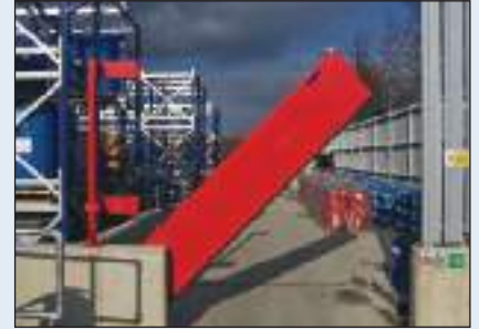
Gas-lift pivot barrier for vehicle access
