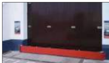
Manual containment barrier for vehicular access
