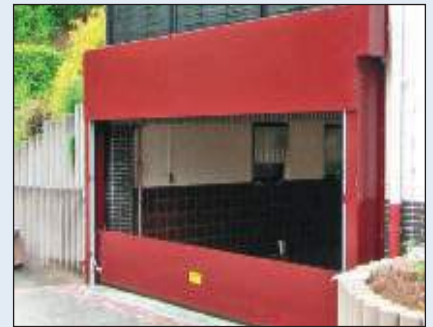
Automatic drop-down barrier
