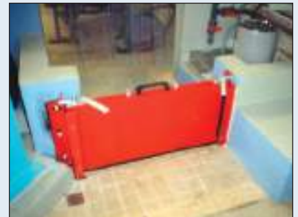
Manual containment barrier for pedestrian access
