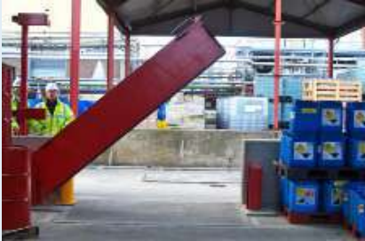
Gas-lift pivot barrier for vehicle access
